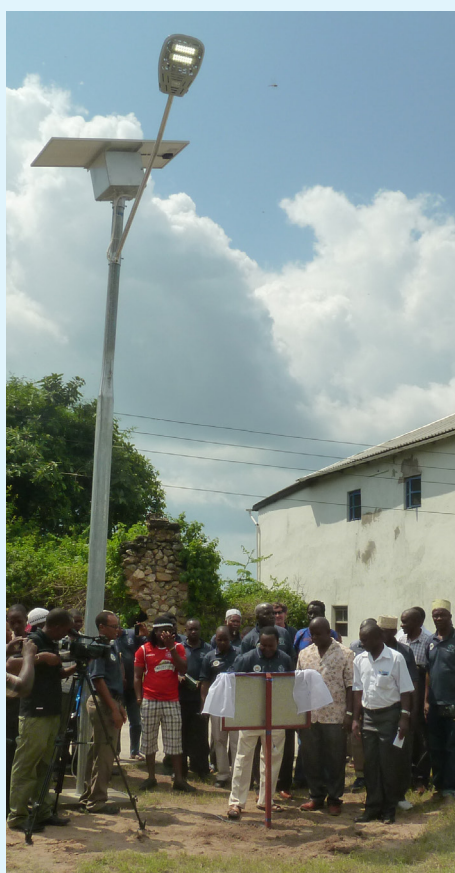
Solar street lamps official commissioning event in the Bagamoyo Demo Site, Tanzania (Photo: COAST Project)
