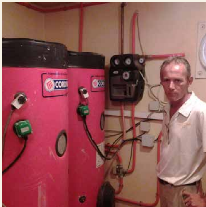
Mr. Martin Schmitz, showcasing the hotel solar water boilers that are used to heat the water in the kitchen and for the laundry services (Photo: COAST Project)
