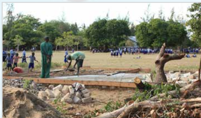
The construction of the platform for the water plant is now complete. The water equipment installation is expected to commence at the earliest opportunity (Photo: COAST Project)
