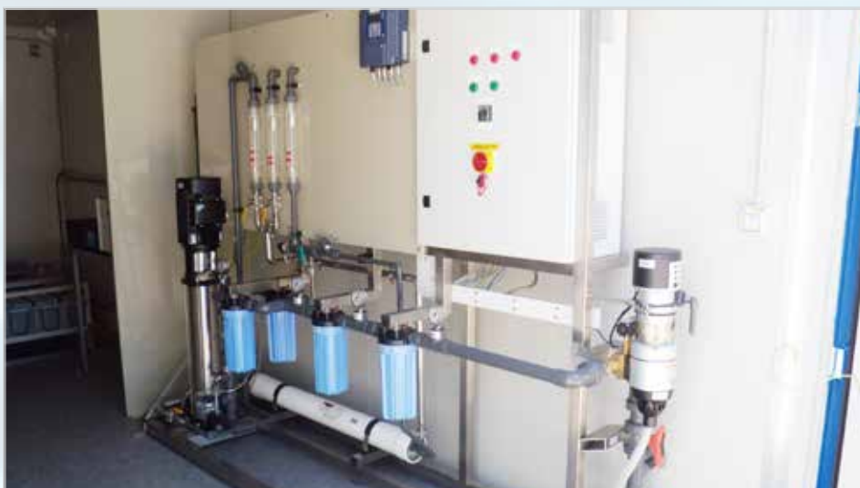
A picture of the water treatment equipment. The equipment utilizes reverse osmosis technology (Photo: COAST Project)
